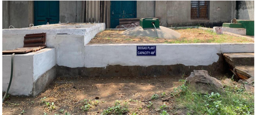
Biogas Plant at Campus
