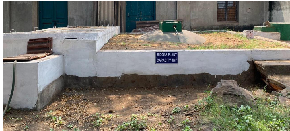
Biogas Plant at Campus
